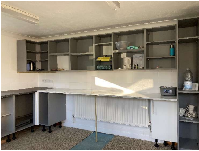
Wall and base units and worktops fitted
