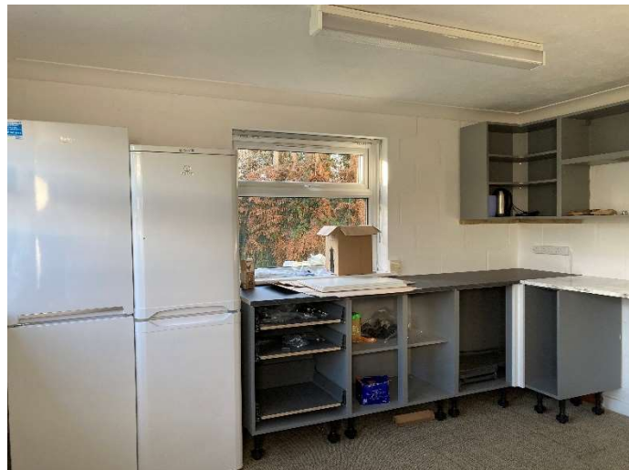
Wall and base units and worktops fitted
