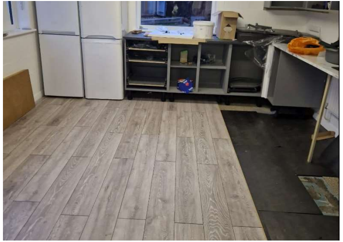
Flooring going down
