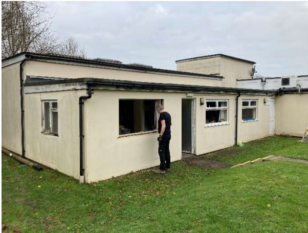
New windows being installed
